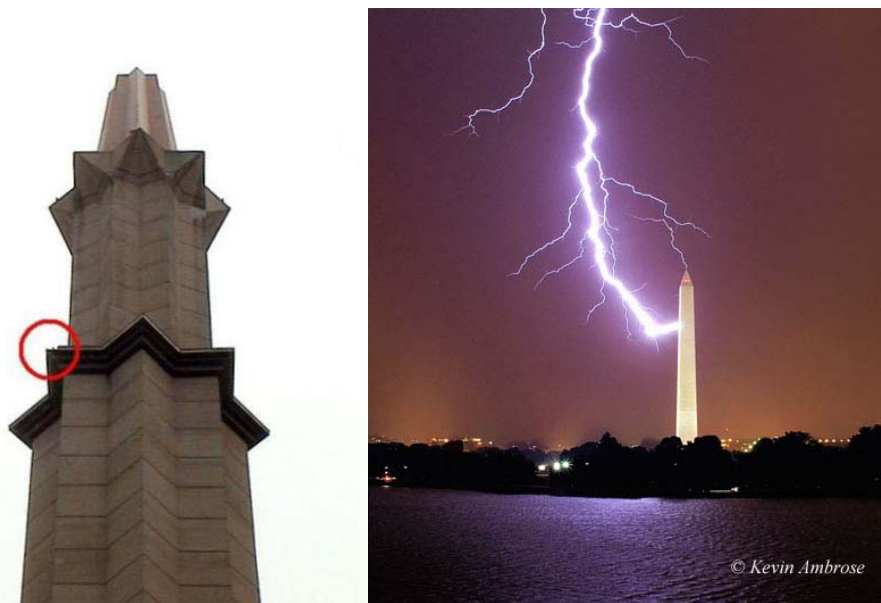
Fig. 8 – The photo on the left shows the location of the bypass on the minaret. The photo of the Washington Monument on the right shows how lightning might have struck the side of the Putrajaya minaret (Courtesy: Kevin Ambrose)
