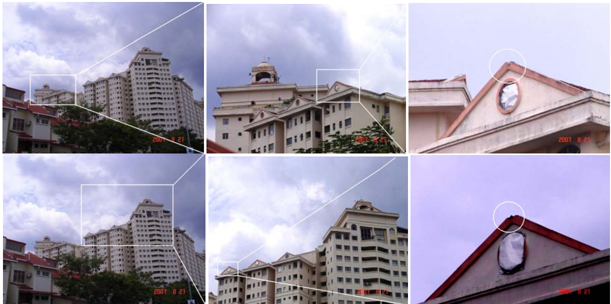
Fig. 6 – The two bypasses that occurred at the northern side of the Crimson Apartments.
