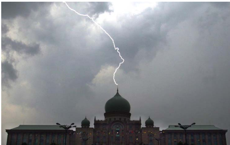
Fig. 12 - A photograph of the return stroke attached to an ESE air terminal (Courtesy: The Star Publications, Malaysia).
