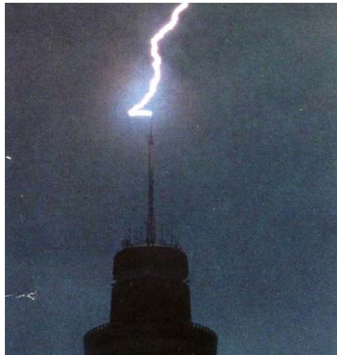
Fig. 11 – A photograph of the return stroke attached to a CVM air terminal (Courtesy: Global Lightning Technologies/Erico).
